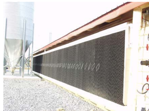
Illustration 1: Typical cool cell seen for broiler houses
